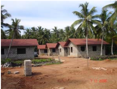
FOLTR Akurala Housing Project
